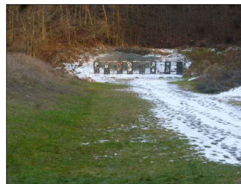
PHOTOGRAPH OF EXISTING 100 YD BACK STOP NO SCALE
